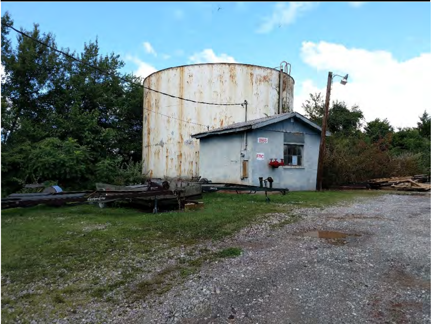
Fire pump building and 10,000-gallon water storage tank
