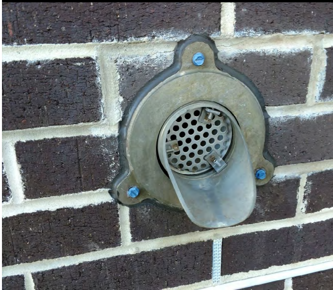
Secondary roof drain nozzle with "after market" rodent/bird nest protection
