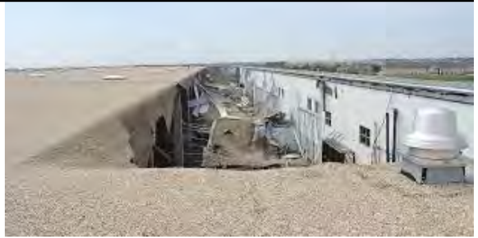
Roof collapse http://rci-online.org/wp-content/uploads/2018-cts-patterson-mehta.pdf
