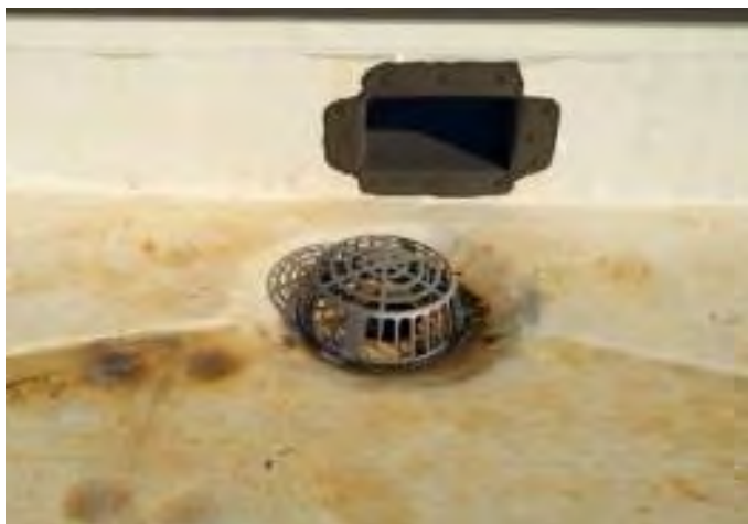
Roof drain & parapet wall scupper
