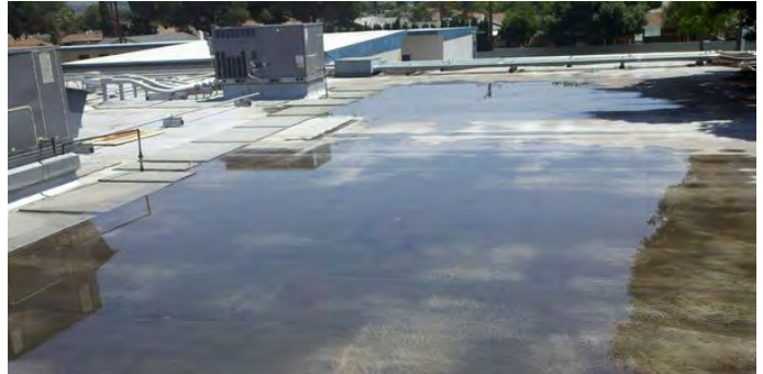
Stormwater ponding https://superiorroofdrainpans.com/common-features
