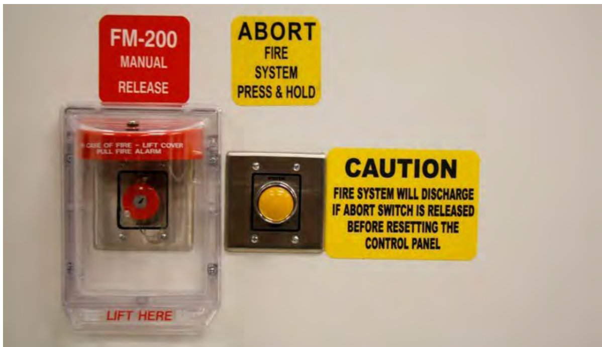
Clean agent manual release and abort switch http://www.aoc.nrao.edu/widar/subsystems/fire/
