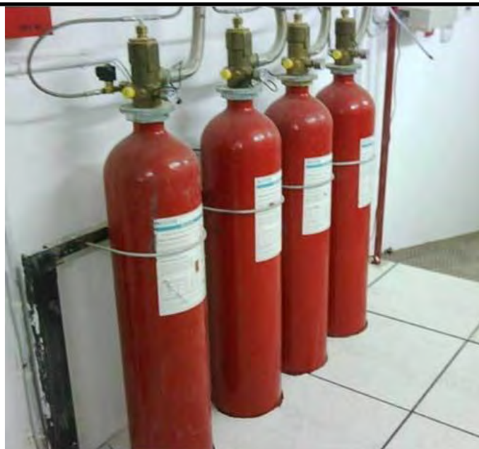
Clean agent gas cylinders https://www.indiamart.com/proddetail/halon-fire-extinguisher-15943312262.html
