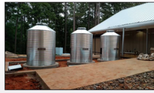
Storage (Above Ground Bolted Steel)
