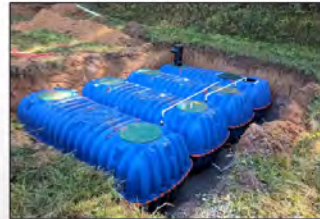
Storage (Below Ground Polyethylene)
