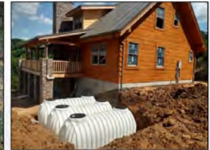
Storage (Below Ground Polyethylene)
