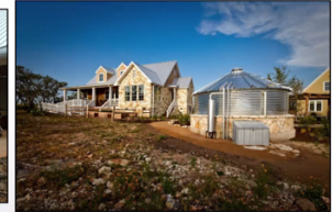
Storage (Above Ground Bolted Steel)
