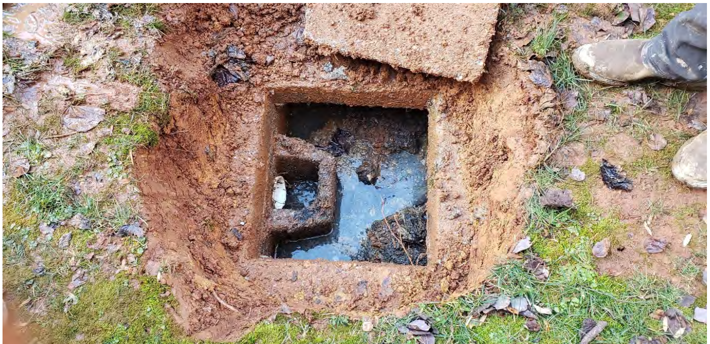
Below: Clogged Septic Tank in Samer's Backyard!
